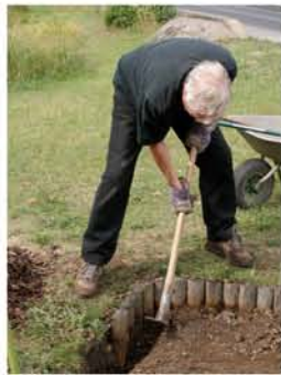
The old rotten logrolls crowbar'd out, and the trench re-dug.
