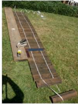
The 156 palings were stapled together onto polypropylene strapping to form six rolls of 26 palings each.
