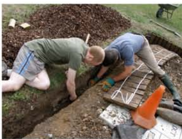
The new logrolls set in, levelled, and back-filled.
