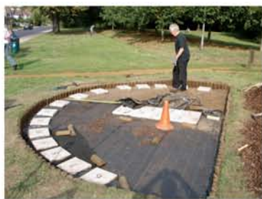
New membrane laid to suppress weed growth, and bark layer replaced. Voila!
